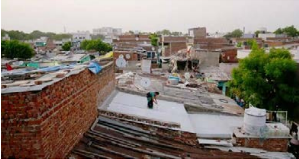
Solar reflective paint being used in Ahmedabad to lower the temperature of houses as part of their Cool Roofs Initiative. Source: Times of India.
